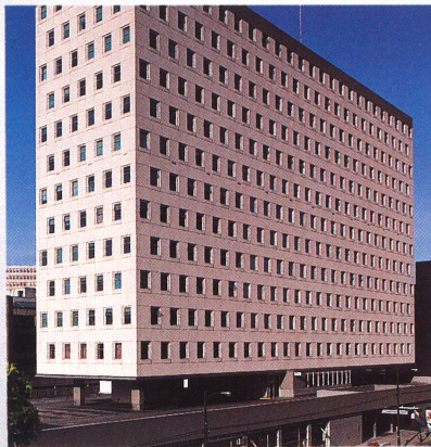
The Fairmont Medical Building 750 West Broadway
